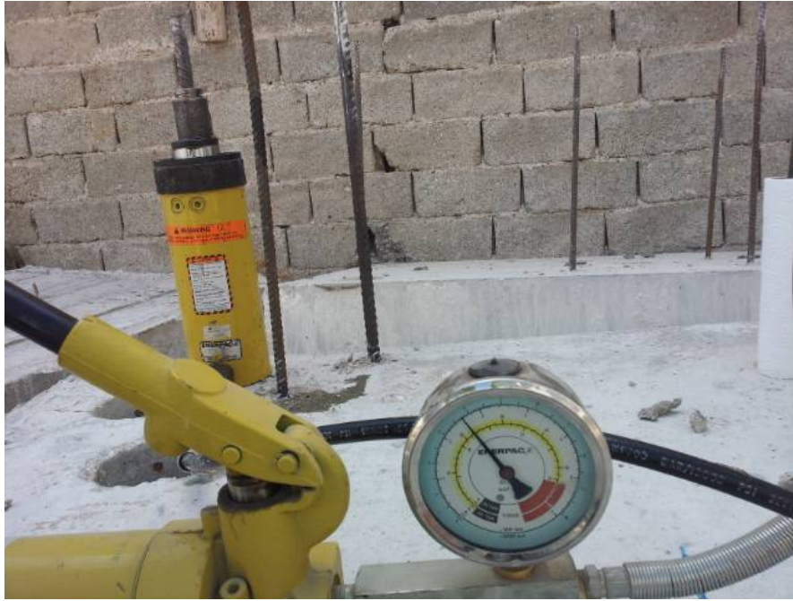
Fig.3. Hydraulic test apparatus of anchor rebar.
