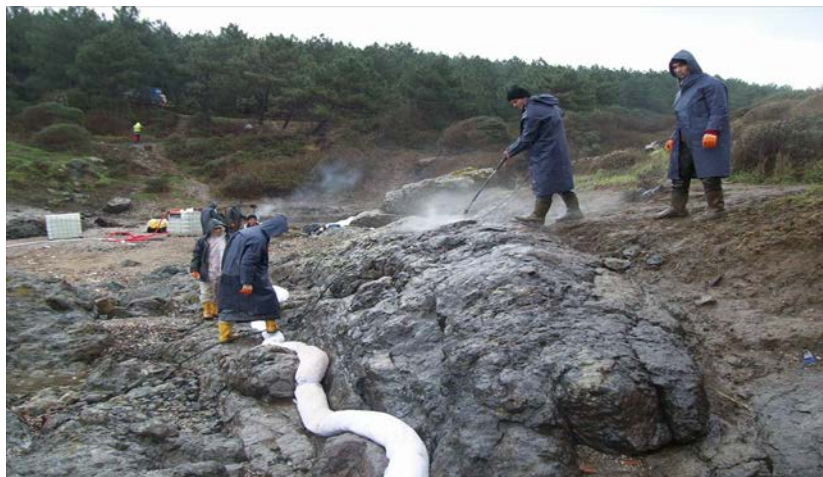
Figure 23. Washing rocks with hot pressurized water
