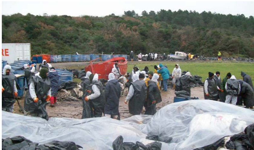
Figure 24. Preparing temporary waste storage area.
