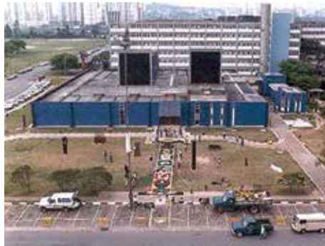
Figure 2.7. Open of the building of MAC at the University City
